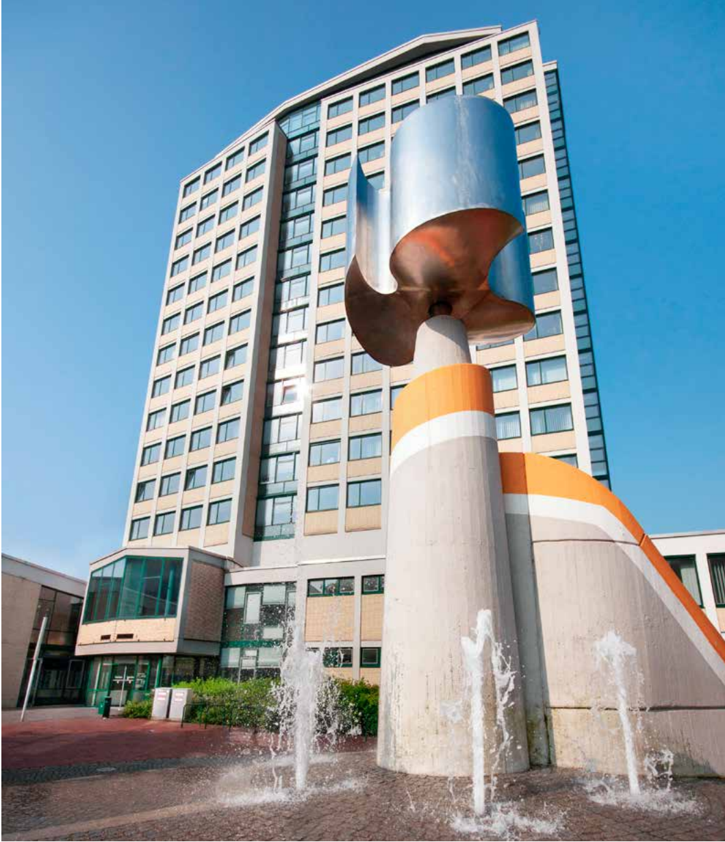
Some 250 smart radiator thermostats have been installed in Lünen's town hall.
